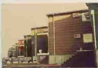
Housing Development, Street View, Jersey City, New Jersey
